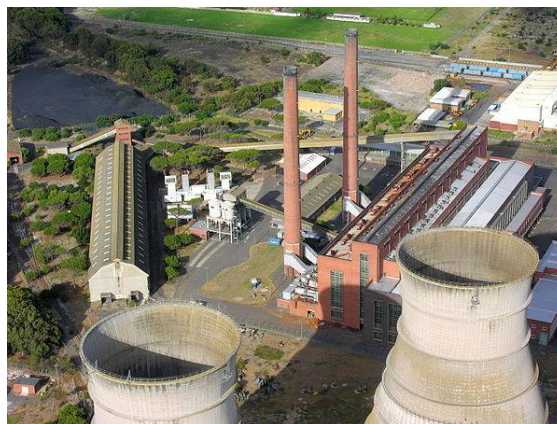
The Athlone Power Station in Cape Town, South Africa.
