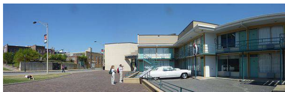
Wide view of the Lorraine Motel and the boarding house from which James Earl Ray fired the fatal shot from a second-floor bathroom window (to the left of the pole).
