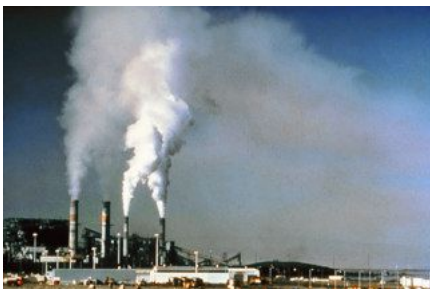
Before flue-gas desulfurization was installed, the air-polluting emissions from this power plant in New Mexico contained excessive amounts of sulfur dioxide
