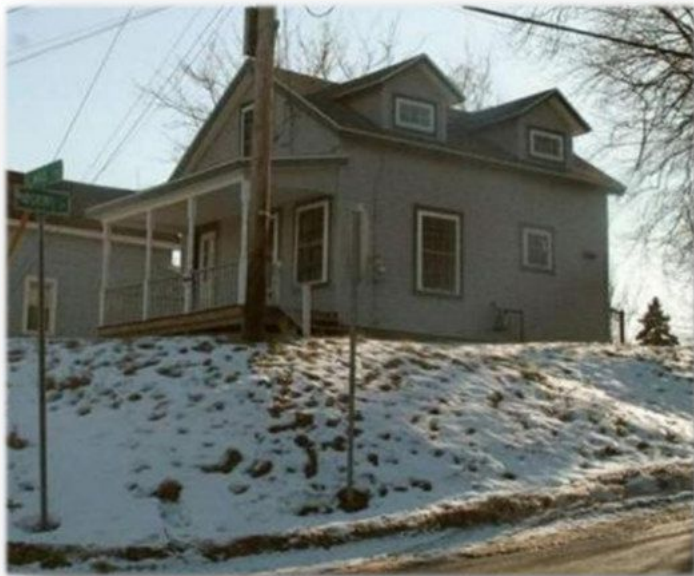
This house cost $105,000 to renovate, but was sold for only $42,000. The city neglected to survey the property prior to the renovation and as a result a driveway could not be added because the house is located on a steep hill.
