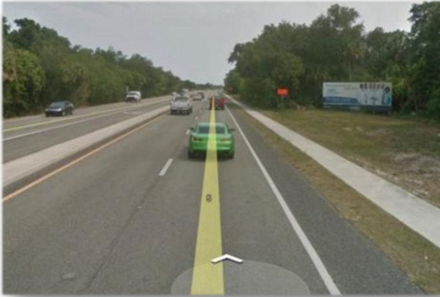
A look at the sidewalk's route with Google Streetview
