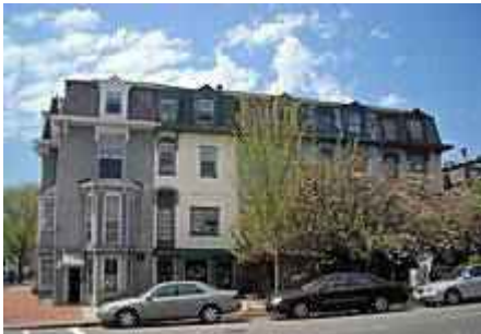
Douglass' former residence in the U Street Corridor of Washington, D.C. He built 2000–2004 17th Street, N.W., in 1875.
