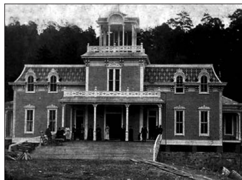
The Ozark Bathhouse in 1880. Go to http://www.nps.gov/hosp to see how the bathhouse looks today.
