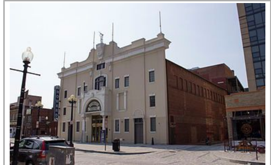
Exterior of theatre after renovation (c.2015)
